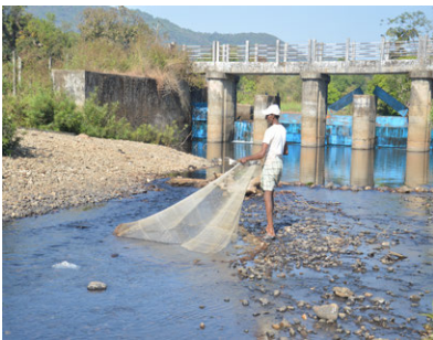
Fig. 11.6: A barrage on Thane stream in the Mhadei
