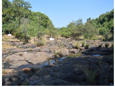
Fig. 11.3: Kalasa stream downstream of irrigation canal leading to disconnected habitat. Haltara dam is proposed here.
